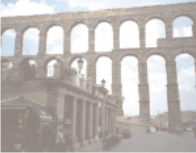
Roman aqueduct near Segovia, Spain still in use today
